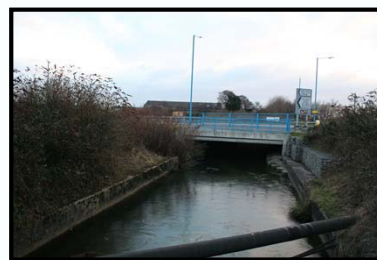
Afan Dock Feeder
